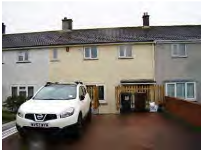
Davis Avenue, Torquay
