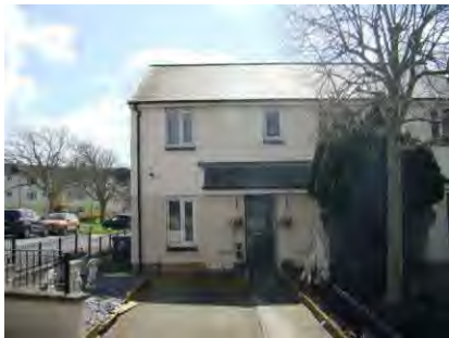
Balfour Terrace, Devonport, Plymouth
