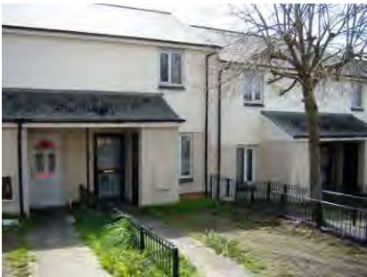
Balfour Terrace, Devonport, Plymouth
