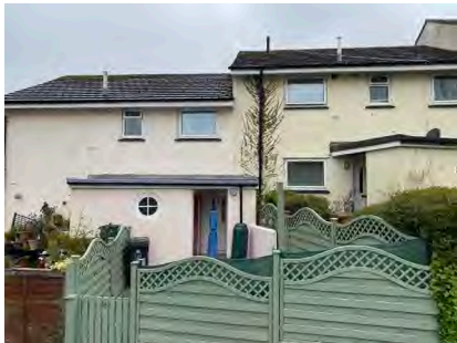
Townsend Close, Kingsbridge
