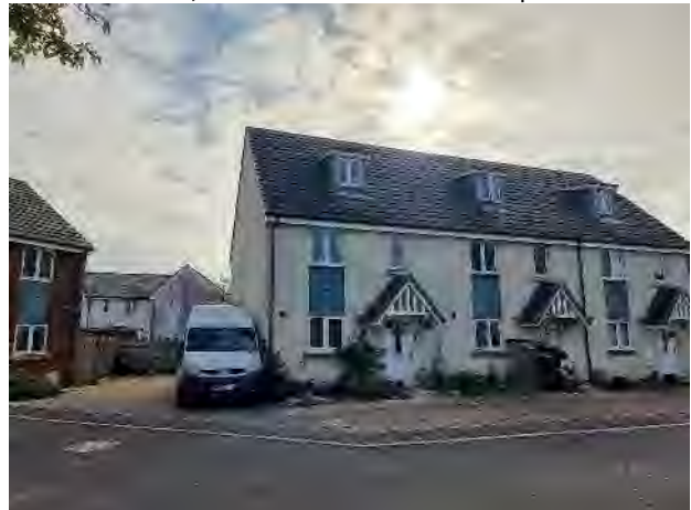
BS24 8EP, 31 Hafner Green WestonsuperMare
