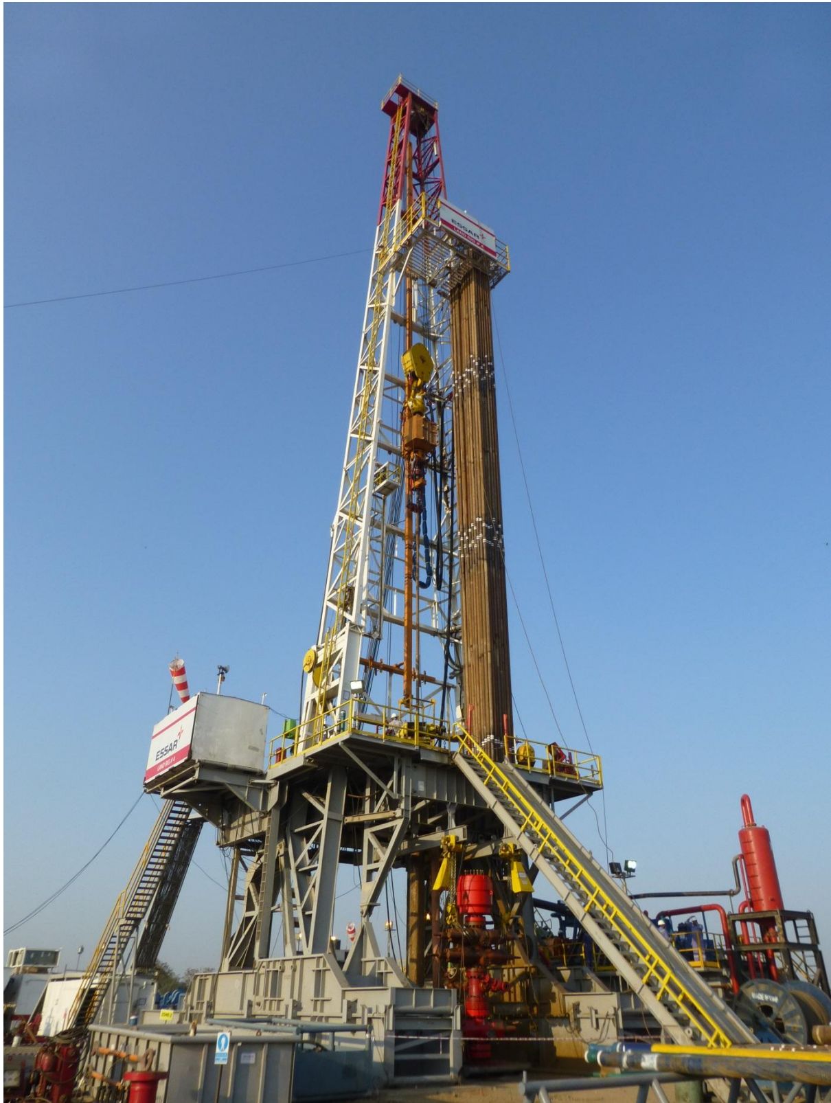
Figure 3: Essar Land Rig 4 at Cambay-77H
