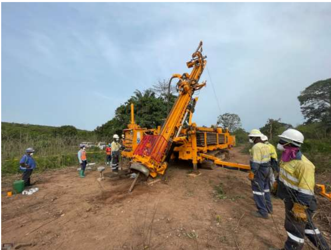
Figure 1: Sandvik DE 810 multipurpose RC drill rig collaring the first hole on site at the Ewoyaa West target.
