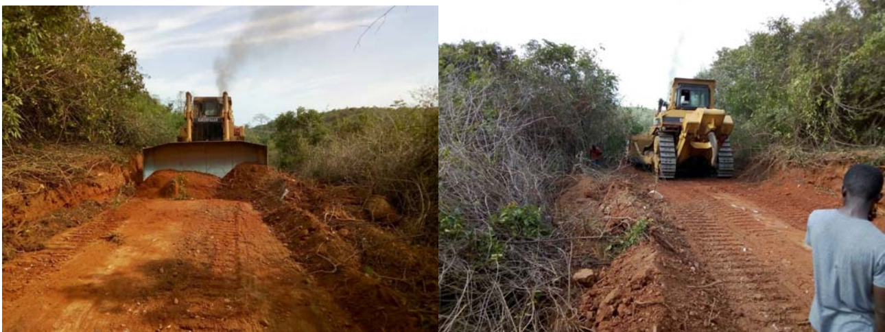
Figure 1 | Bull dozer commencing earthworks for drill access at the Ewoyaa pegmatite target
