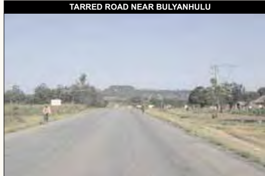
TARRED ROAD NEAR BULYANHULU
