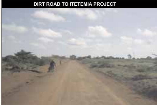
DIRT ROAD TO ITETEMIA PROJECT
