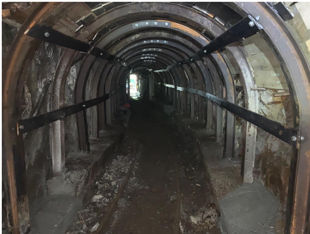
Figure 5: Completed Llechfraith Adit Repair
