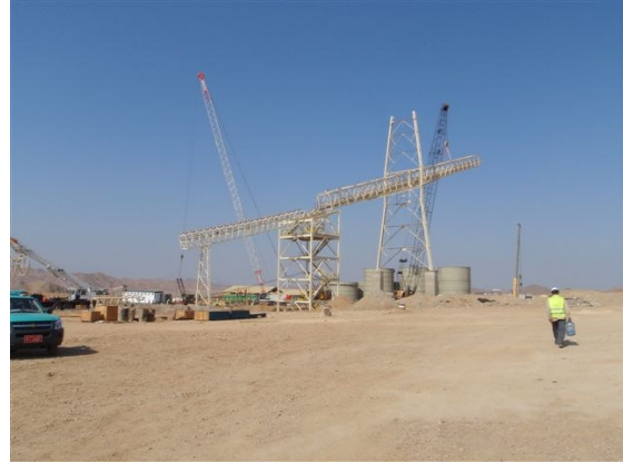
Progress Pictures: Power station footings and structural steel in the background (left) and Conveyor 01 (right)
