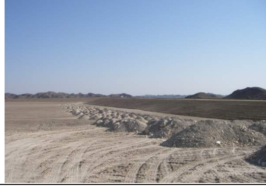
Progress Pictures: Tailings Storage Facility: Completed Embankment (left) and Gypsum lining for Embankment Face (right)
