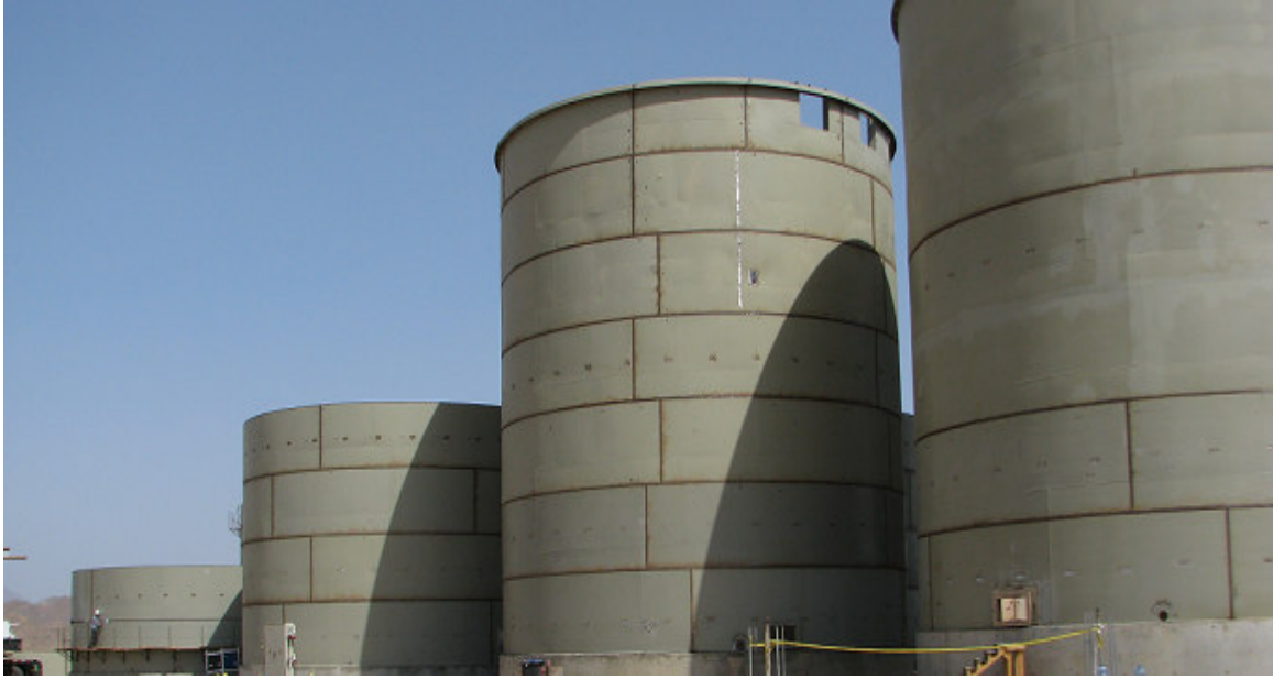
Progress Picture: Tank Construction
