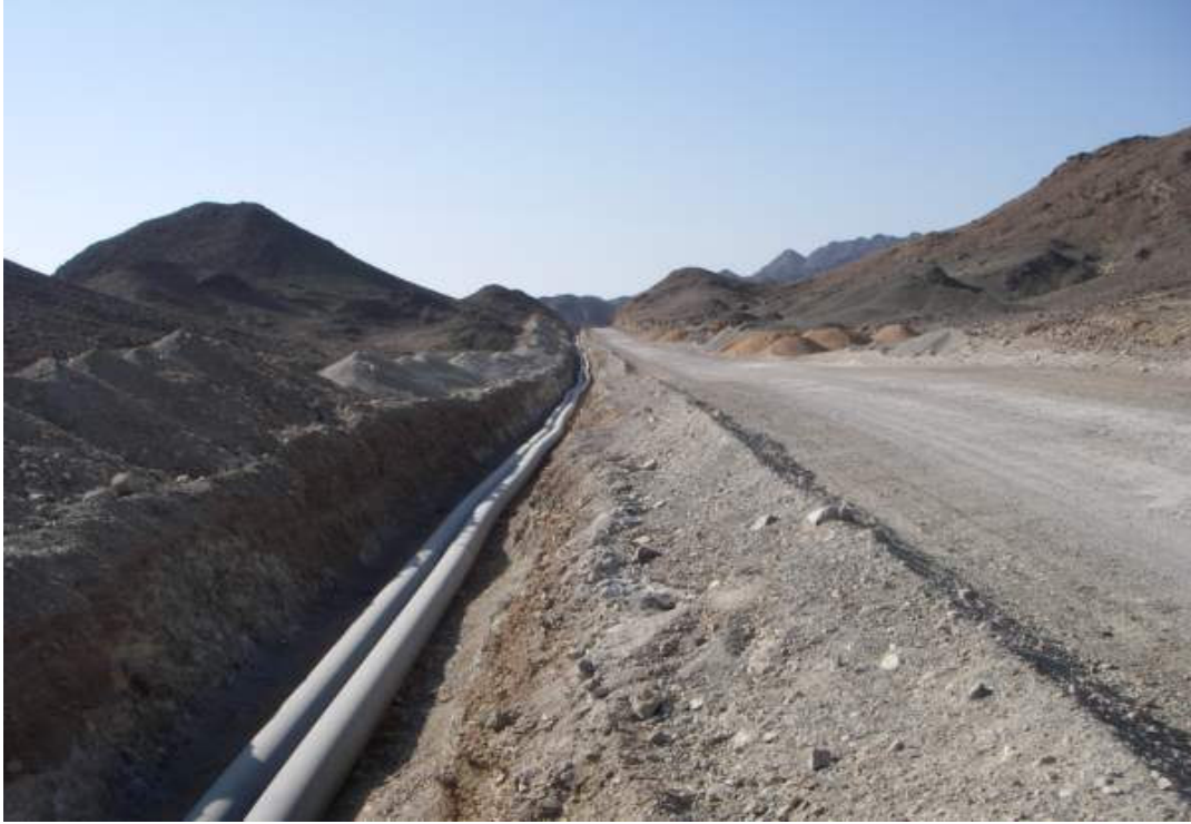
Progress Picture: Seawater Pipeline in place prior to backfilling of earthworks
