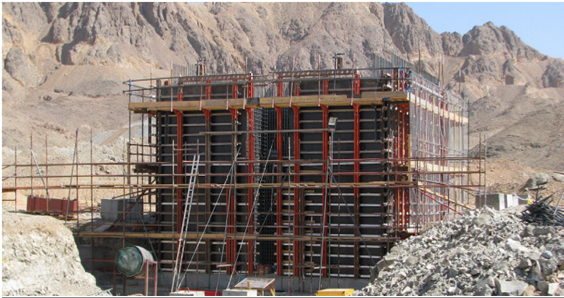
Progress Picture: Primary Crusher foundations under construction
