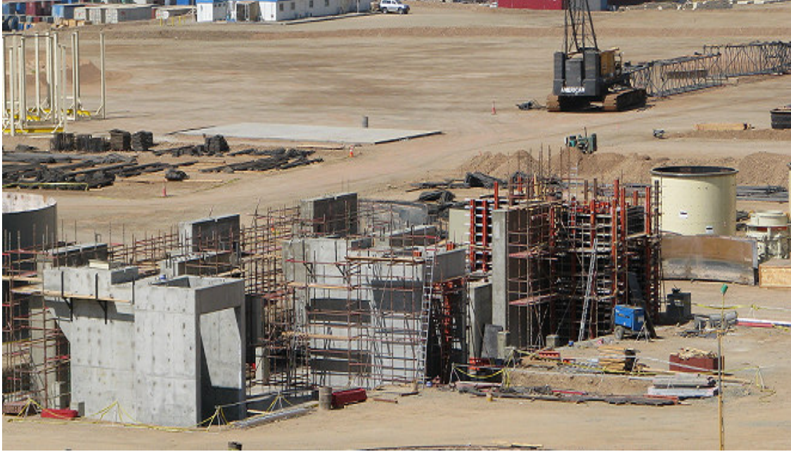
Progress Picture: SAG Mill pedestals and Motor/Pinion slabs under construction
