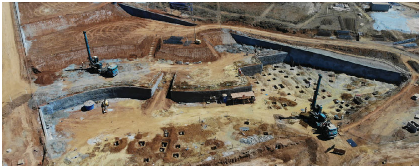
Bento Rodrigues school construction works.
