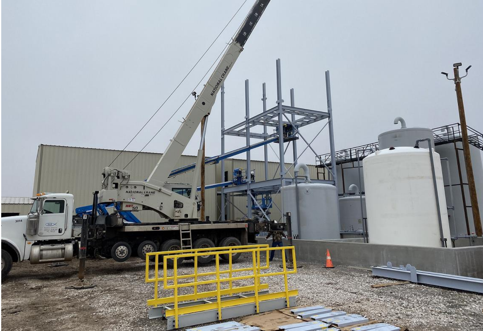
Figure 1. Construction of IO#8 in western Oklahoma
