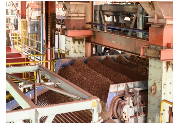
6 MTPA pellet plant commissioned at TSK
