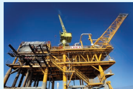
Above: LAM A platform in the Dzeheitune (LAM) field.
