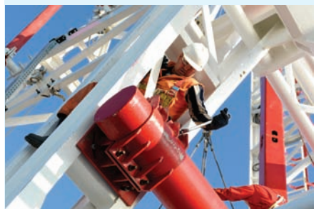
Above: Drilling operation.
