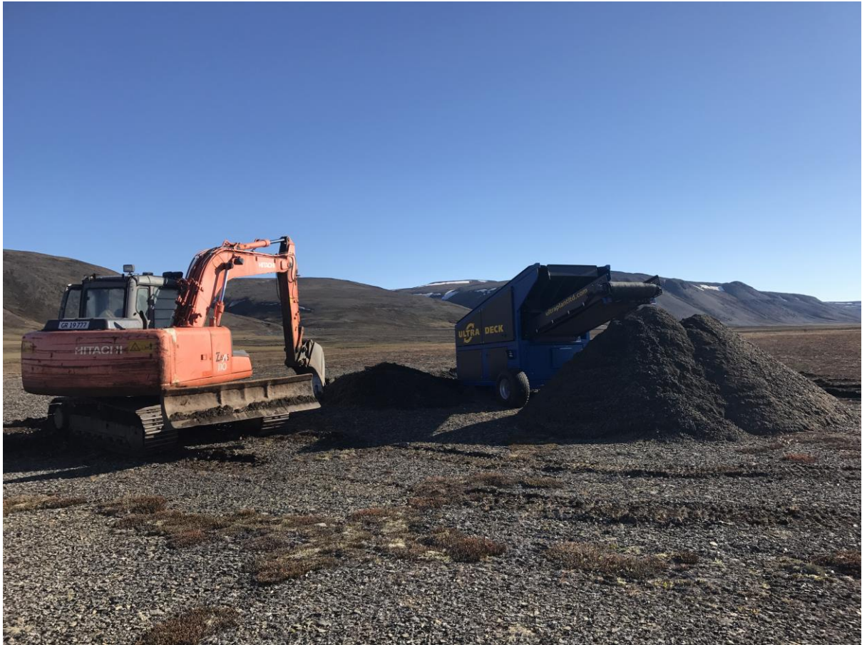
Figure 5. Stockpiling commences of sorted high grade ilmenite concentrate
